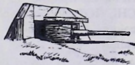
Six-inch Mark VII gun with concrete hood 1942-1946
